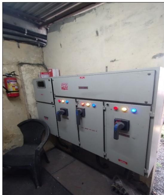
Fig 4.12. Plastic chairs, cardboard boxes, and scrap materials such as old SFUs were found stored inside the electrical room, which is a violation of standard housekeeping and safety practices.
