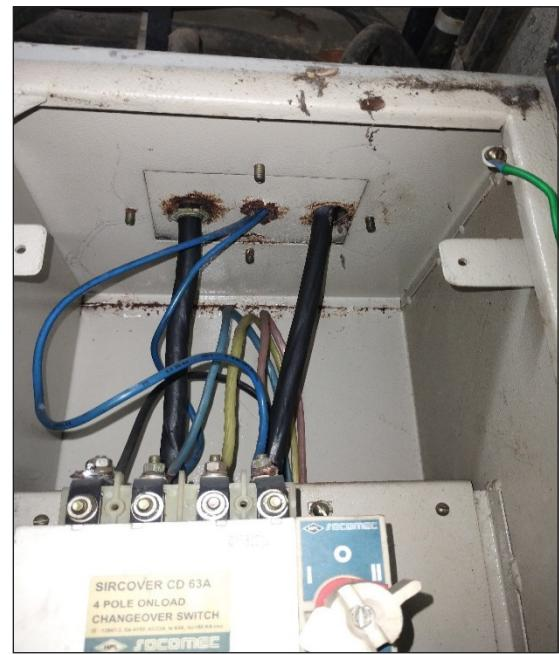
Fig 4.18. Multiple cables were found entering the TO VDB-4 panel (Economics Block) without proper cable glands or sealing arrangements, resulting in potential damage to the cables due to sharp
