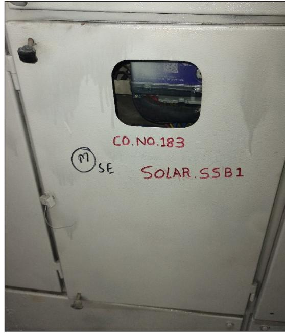
Fig 4.14. Multiple meter panels were found without glass covers, which compromises equipment protection and poses a safety hazard.
