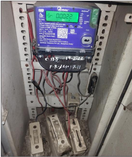
Fig 4.13. Multiple meter panels were found with heavy dust accumulation, indicating inadequate maintenance and posing potential operational and safety risks.
