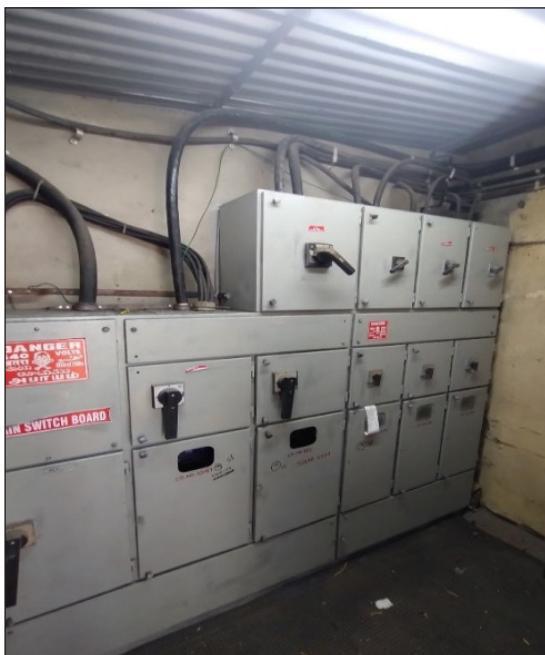
Fig 4.11. Multiple electrical panels were found without proper identification labels indicating their name and rating, which is not in accordance with standard electrical labeling practices.
