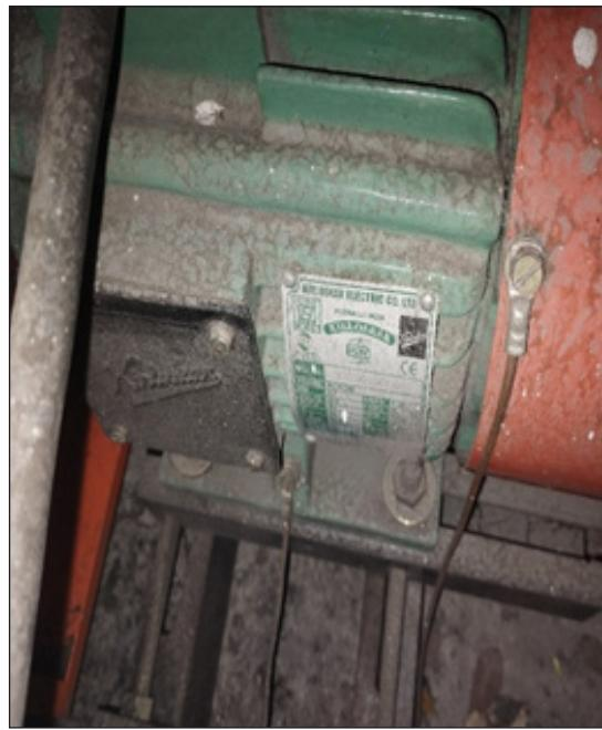
Fig 4.7. Each three-phase motor is equipped with dual earthing points in accordance with standard grounding requirements to enhance safety and fault clearance reliability.
