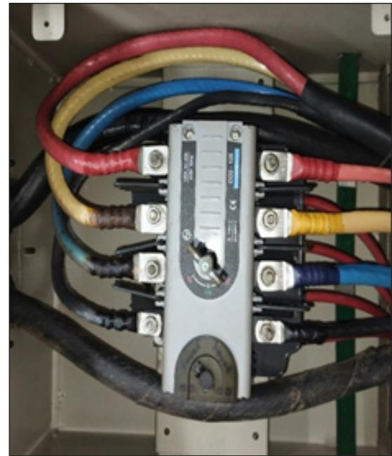
Fig 4.20. Discoloration due to overheating was observed at the cable terminals in multiple panels, indicating possible loose connections or overloading.
