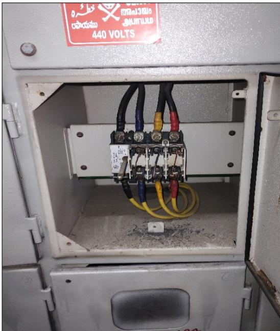
Fig 4.15. Multiple SFUs were found bypassed, indicating a critical lapse in circuit protection and non-compliance with standard electrical safety practices.
