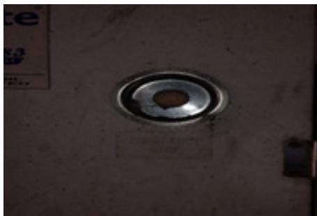
Fig 4.8. An emergency stop push-button is provided for the Diesel Generator (DG) system, facilitating immediate shutdown in case of operational hazards or emergency conditions.
