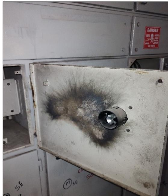
Fig 4.16. Burn marks caused by blown SFUs were observed in multiple panels, indicating past fault incidents and insufficient maintenance or timely replacement.
