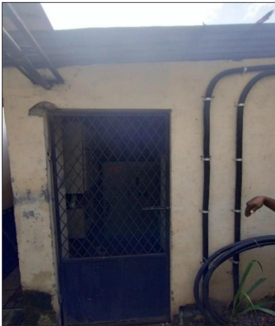
Fig 4.9. The electrical room entrance lacks a visible 'Authorized Personnel Only' signage, which is essential for restricting unauthorized access and ensuring compliance with safety
