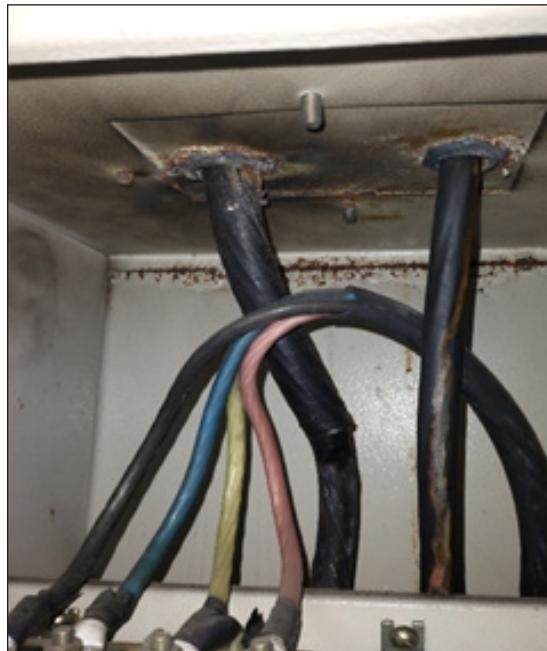
Fig 4.19. Damage to the armored cable due to rusting and signs of overheating was observed inside the TO VDB-3 panel (IGNOU Block), indicating prolonged exposure to moisture and thermal stress.
