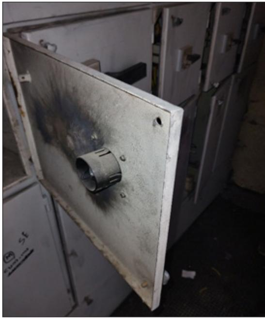
Fig 4.17. Multiple panels were found without rubber door seals, compromising protection against dust, moisture, and ingress, and reducing the effectiveness of the panel's IP rating.
