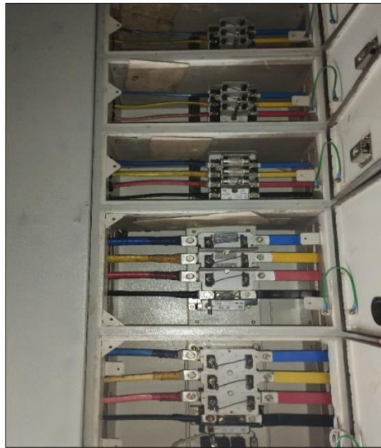
Fig 4.10. All Switch Fuse Units (SFUs) in the DG panels were found electrically bypassed, rendering the overcurrent protection mechanism inoperative and posing a
