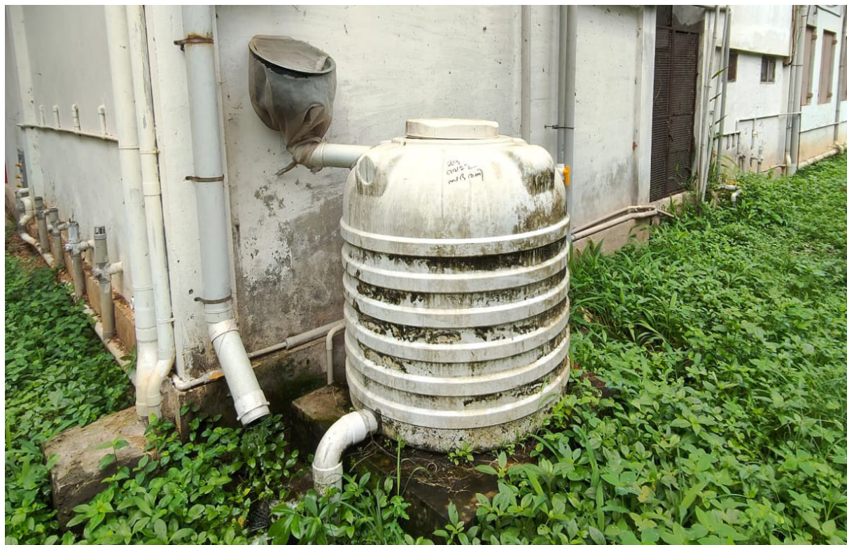
Fig 5.2 Rainwater harvesting system
