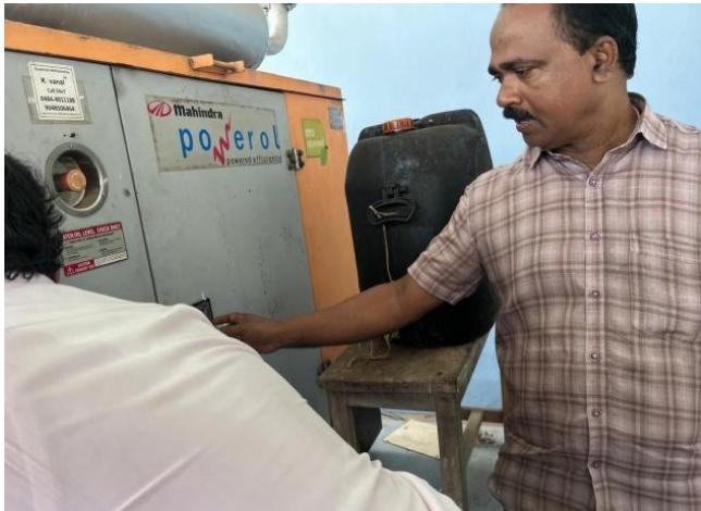
Fig. 4.23 Diesel can kept at the door of DG which will block the access to DG set and cause fire
