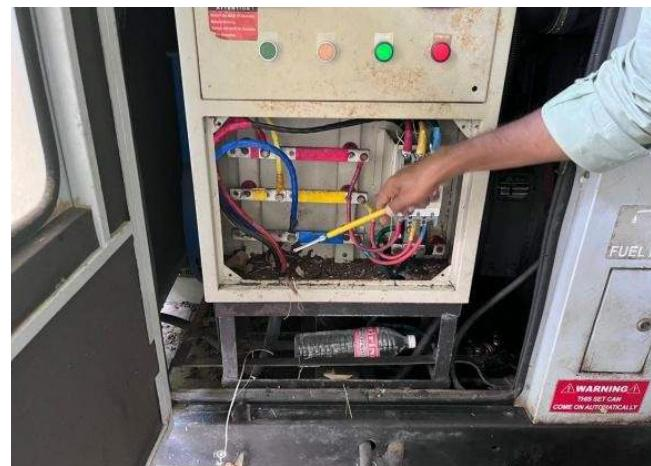
Fig. 4.22 Waste materials present on BUS of DG set
