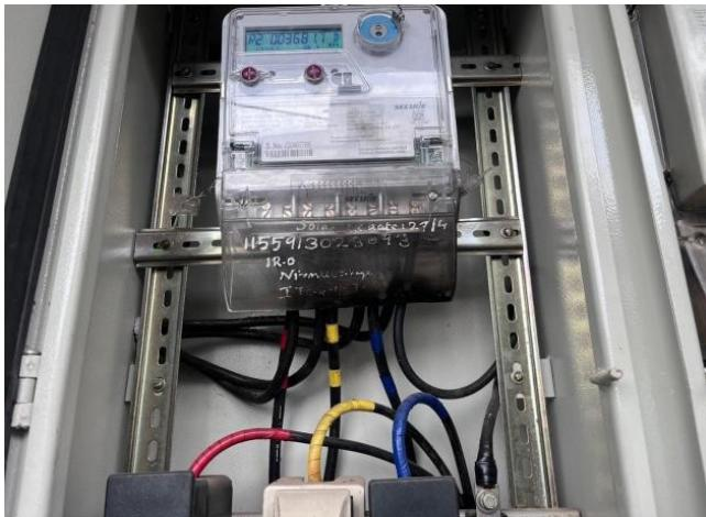
Fig. 4.29 Cables are burned and damages found in KSEBL
