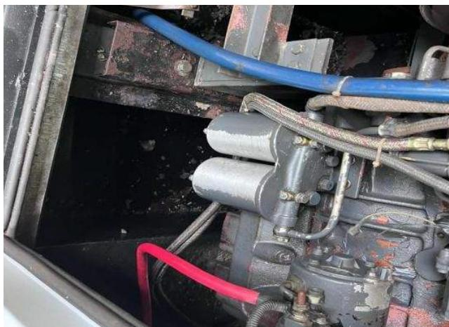
Fig. 4.21 Oil spillage is present inside the DG set
