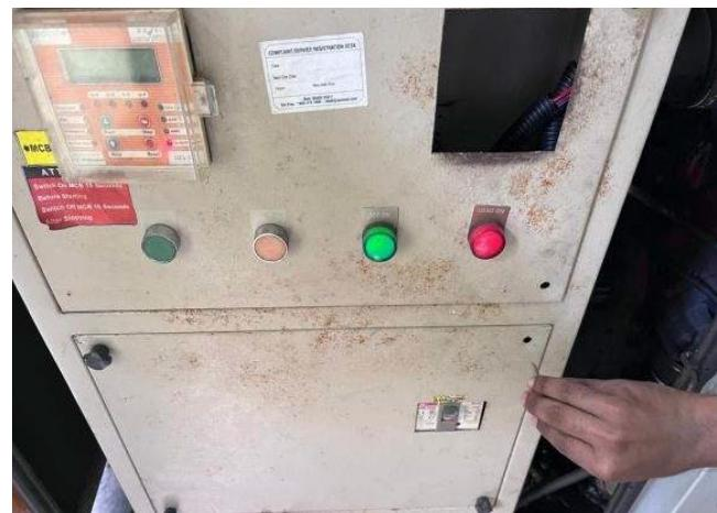
Fig. 4.20 Energy meter are absent in DG GCP
