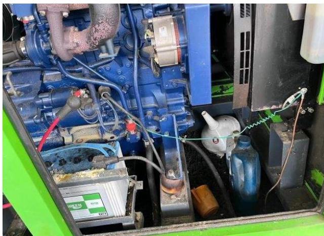
Fig. 4.19 Oil filling equipment are kept inside the DG
