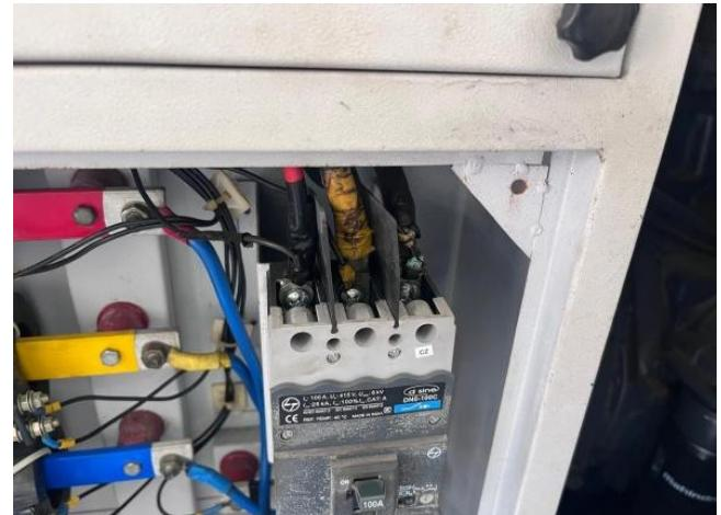
Fig. 4.24 Cable leg of MCCB is burned at GECP
