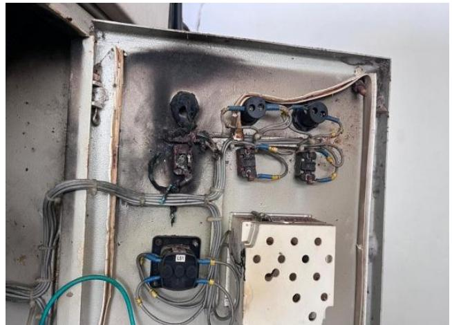
Fig. 4.30 Panel board is burned and running without any protection
