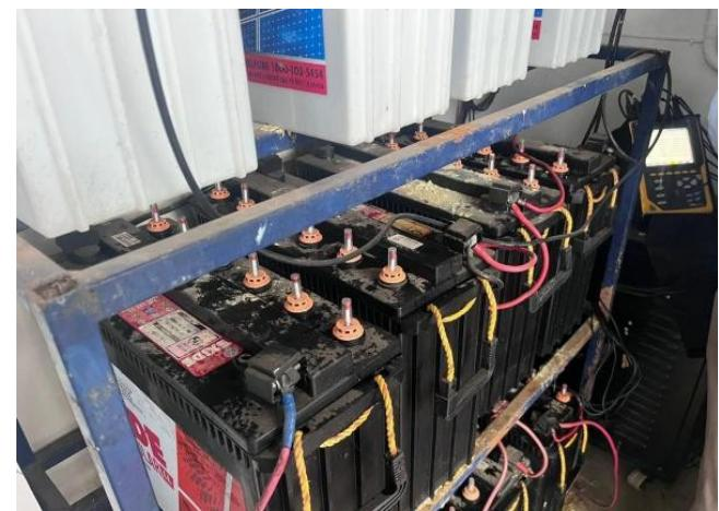
Fig. 4.28 Battery water are spilled out from battery unit
