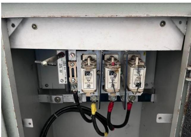
Fig. 4.33 Blown fuses are wired without non-standard bare coper
