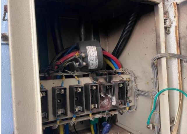
Fig. 4.31Panels are running without fuse links
