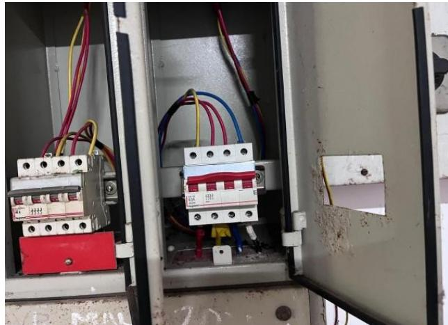
Fig. 4.25 Multiple connections are wired from same switches
