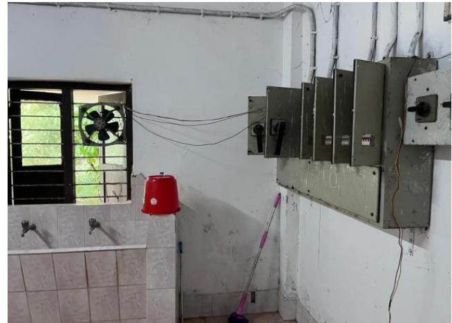
Fig. 4.26 Temprory extension from panel without switch
