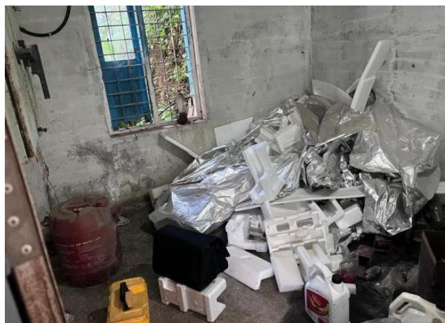
Fig. 4.27 Inflammable materials kept at electric room
