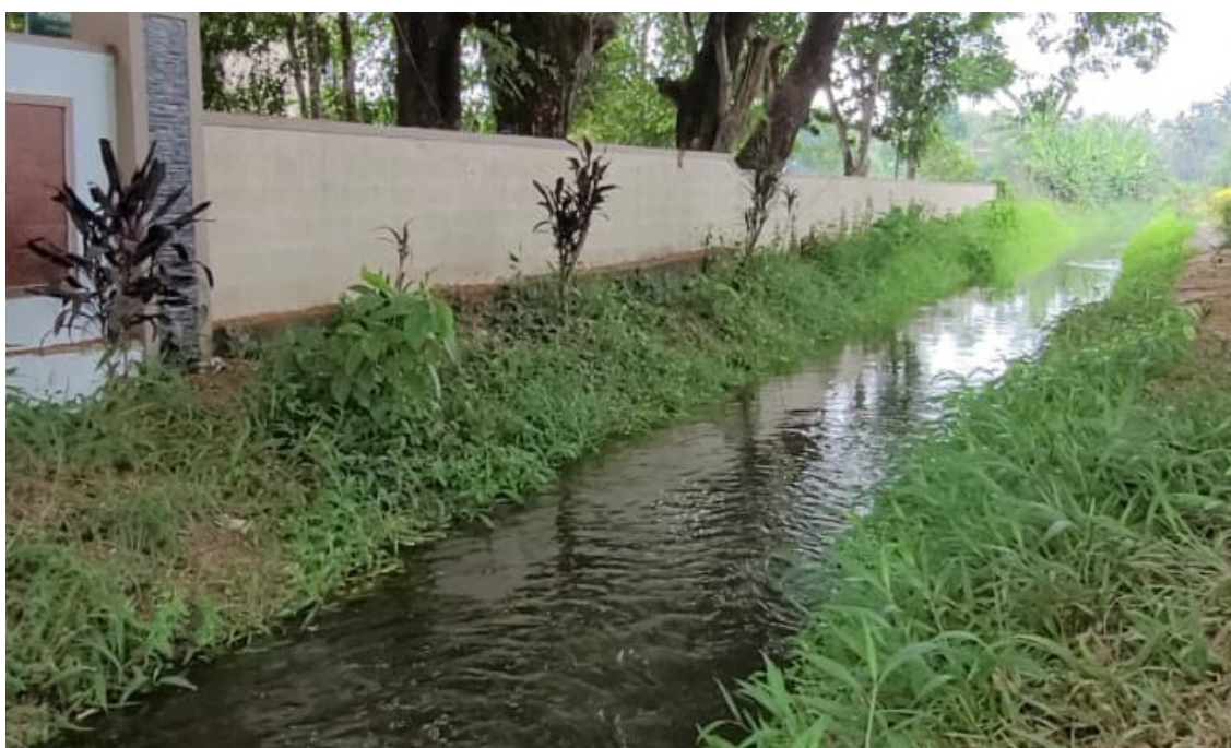
Fig 5.4 Periyar River Valley Irrigation Canal Perumbavoor
