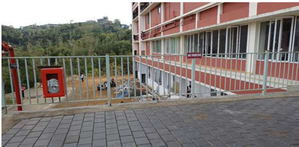
Fig 8.13 Wall-falling and pedestrian safety facilities
