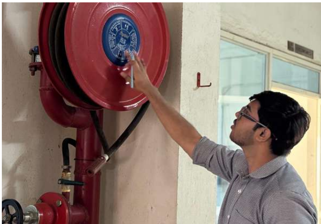
Fig 8.1 Hazards identification and risk assessment - cafeteria
