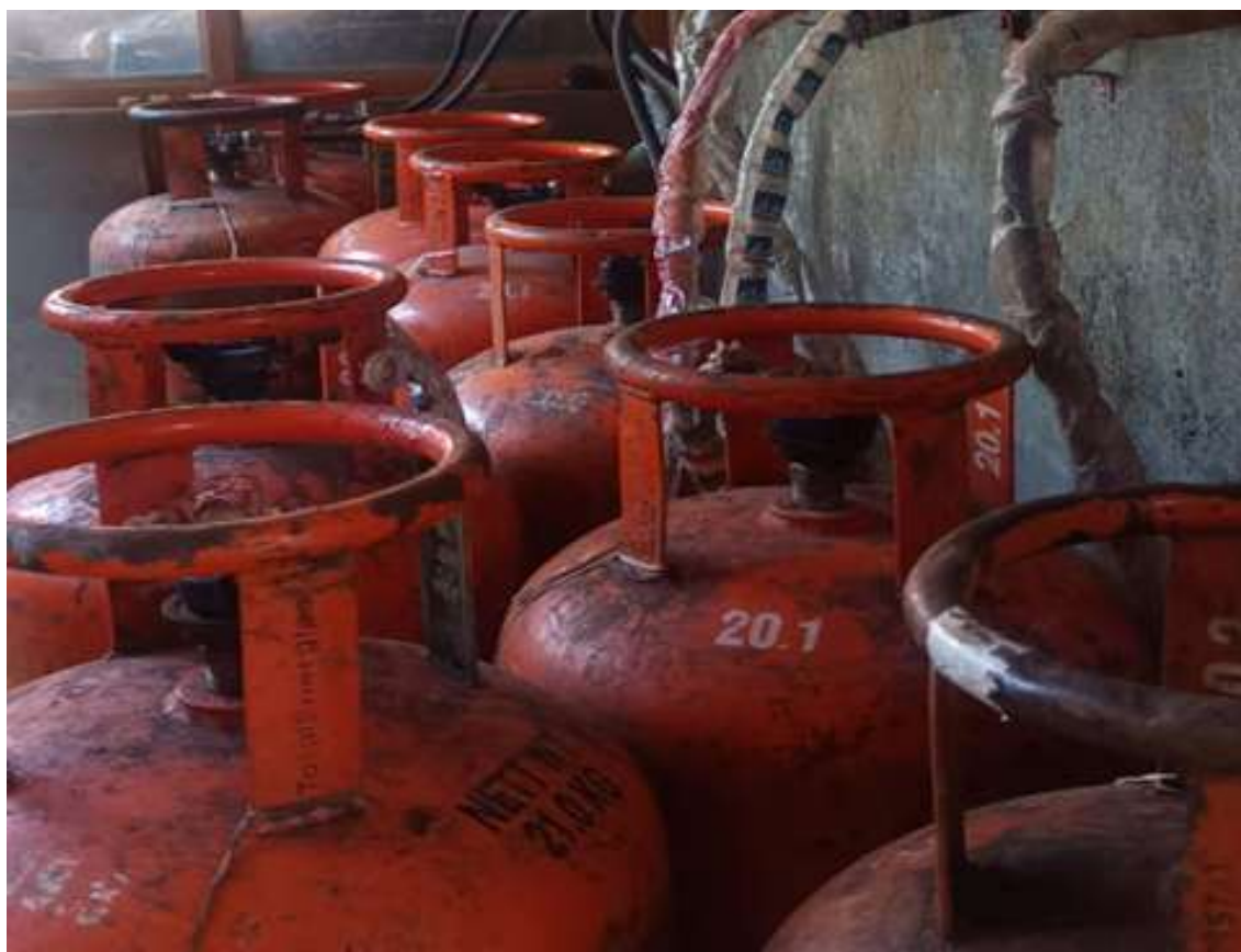
Fig 4.32 LPG Cylinder Supply and Distribution Pattern for College Mess and Canteen
