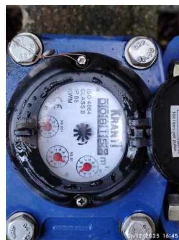
Fig 5.11 Flow water meter reading data collection process
