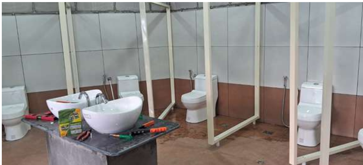
Figure 14. Installation of partition boards began
