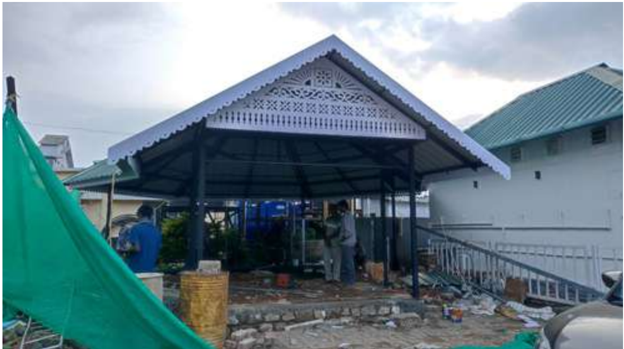
Figure 10. Truss work completed
