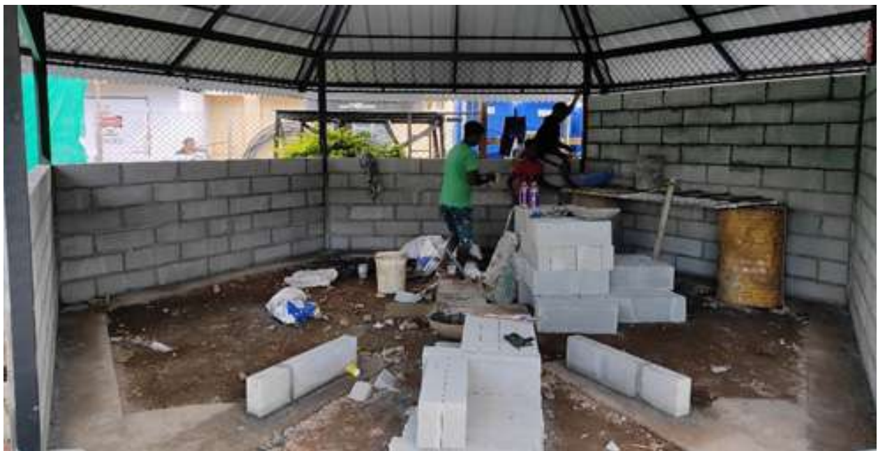
Figure 11. Side wall construction
